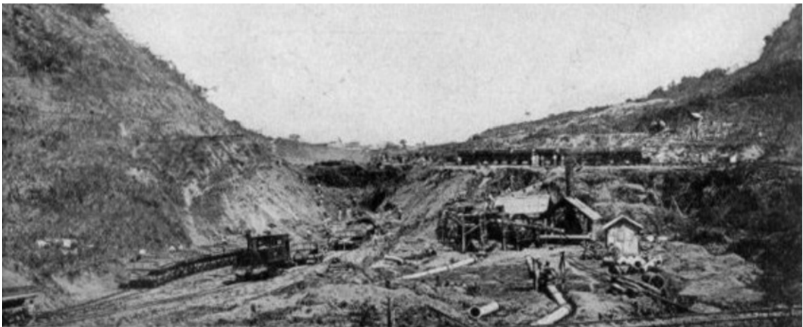
Figure 1 French canal excavation work at Cucaracha, 1885
