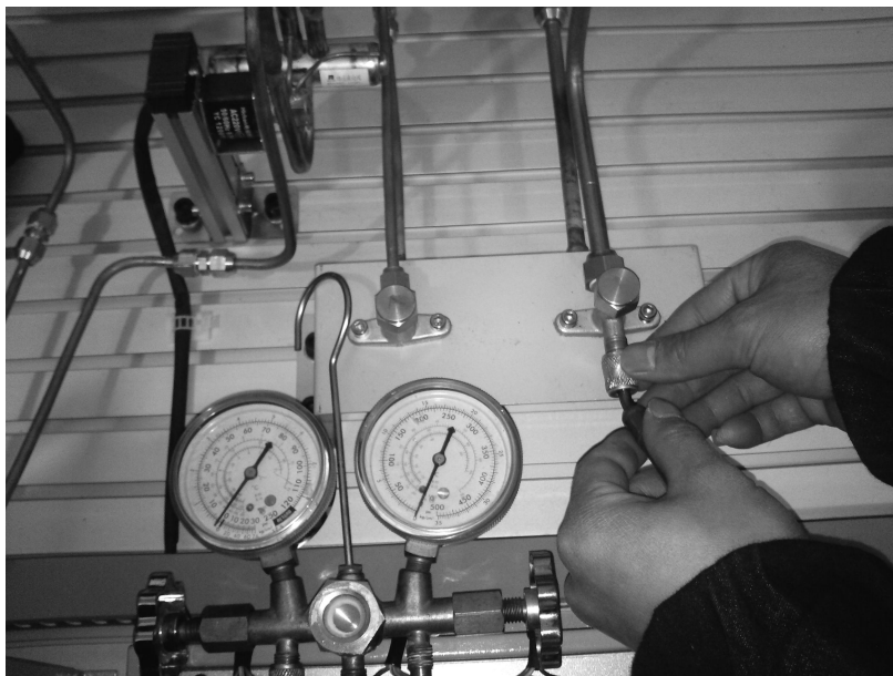
Figure 3-56 Schematic diagram of the air conditioner refrigeration system removing the liquid filling pipe connected to the liquid filling port
