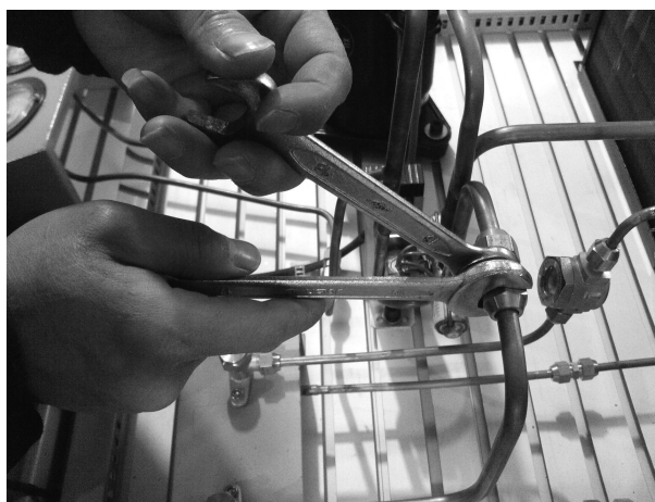
Figure 3-35 Tightening diagram after pipe connection
